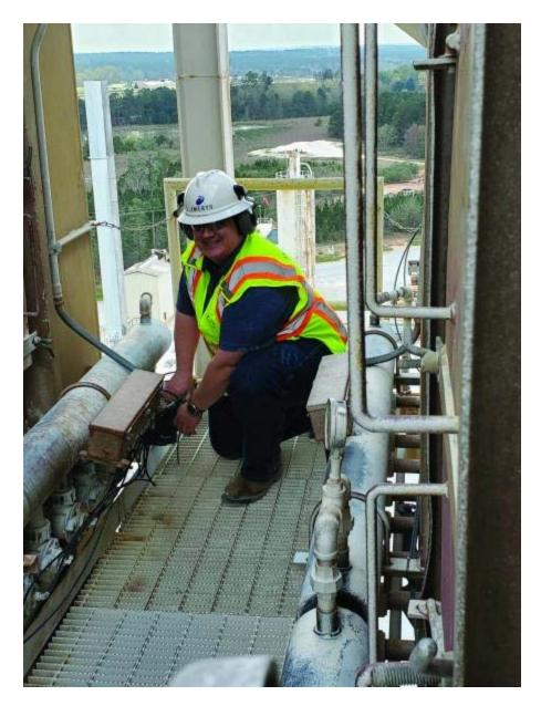
Robin Davis of Imerys Performance Mineral Americas installs a technically advanced pulse valve that has proven to improve dust collector performance and reduce compressed air consumption.
